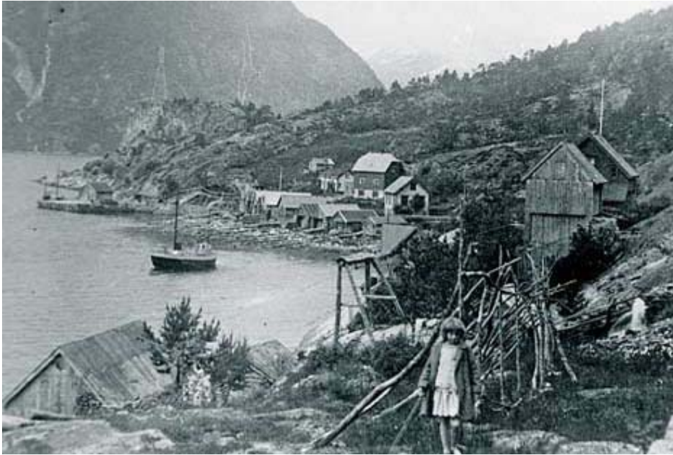
The Fjørå community before and after the 1934 Tafjord accident (3 million m 3 rockslide → tsunami)
