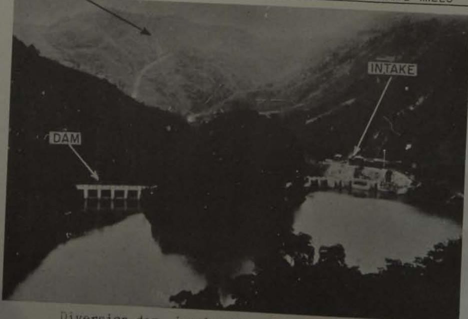
Diversion dam, intake and reservoir at Bukai. Water from this reservoir is carried by tunnel to Lake Jitsugetsutan, 15 miles to the SW. Two small hydroelectric plants were projected NE of here, but their present status is unknown.
