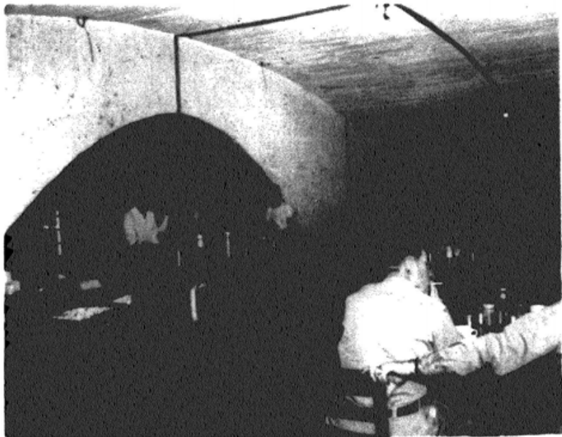
Interior View of Mess Hall.
