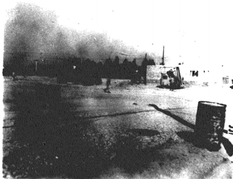
Construction of Roads at Tainan by Army Personnel.
