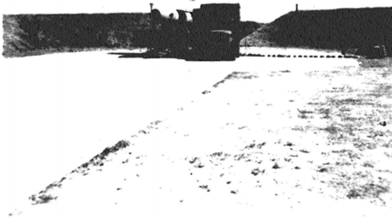
Launching Pads, Tainan Air Base.
